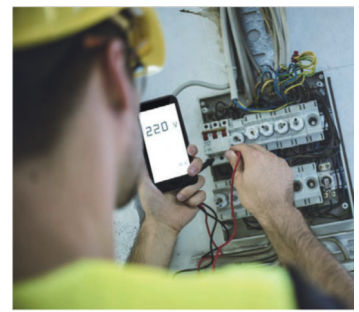
Electric Power Inspection
